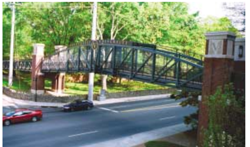
Pedestrian bridge across 21st Avenue S. linking John F. Kennedy Center to MRB III
